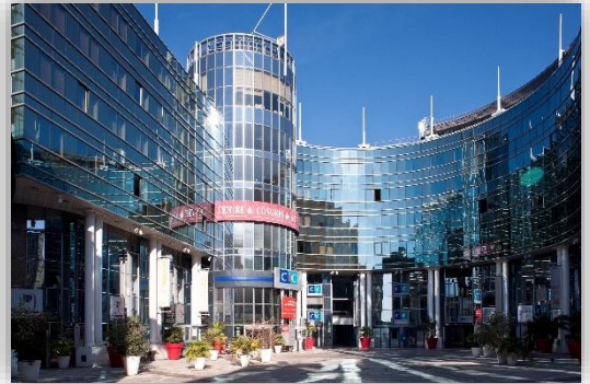
Convention Center – Cité Mondiale 370 m 2 - Central location – Auditorium 300 places
