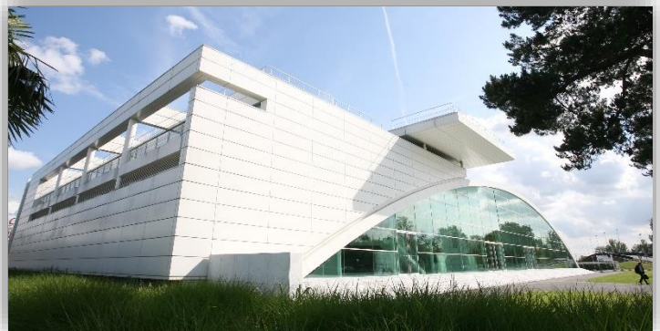
Bordeaux Convention Center 12 000 m 2 - 3 Free visitors parking – Delivery parking – Loading dock – Facing the lake
